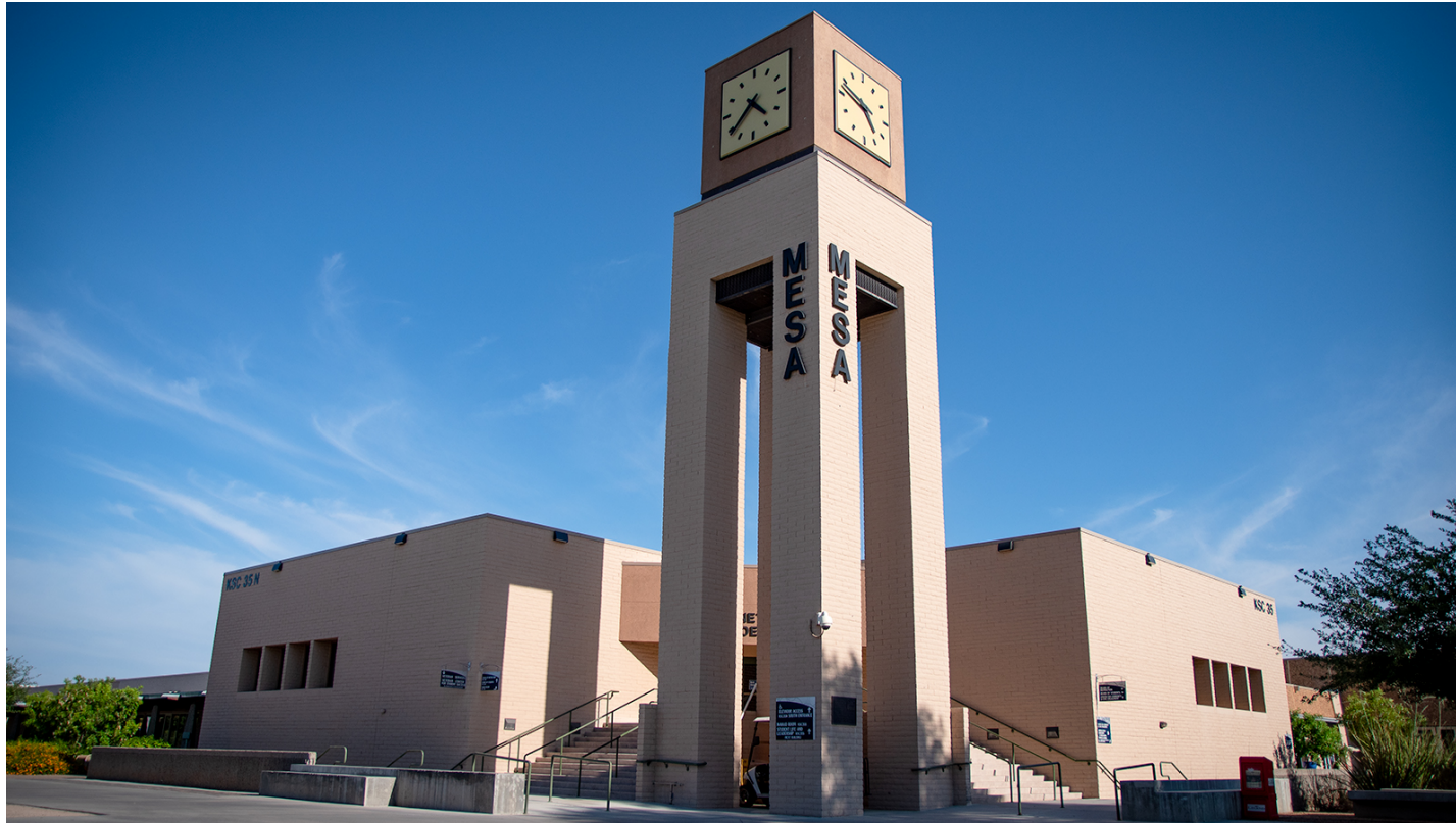
The clocktower in the center of campus at the Southern and Dobson location of Mesa Community College. (Photo by Monica Spencer)
